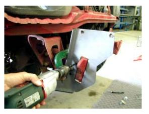
17 Using 10mm holes in the side of chassis bracket as a template, drill out though one side of chassis using 10mm drill bit.
