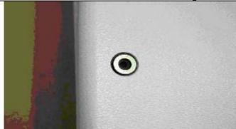
Apply a silicone bead to lower corner of Dia 25mm holes cut into the canopy shell.
